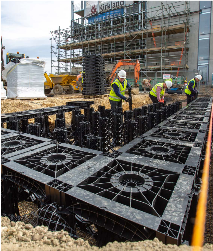
A typical RootSpace installation.
