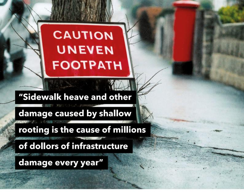
If soil alone is depended on as a structural material and required for the load-bearing of buildings, vehicles, and pedestrians; it will be compacted to the point that air and water are excluded and a totally insufficient space for root growth will be available.
