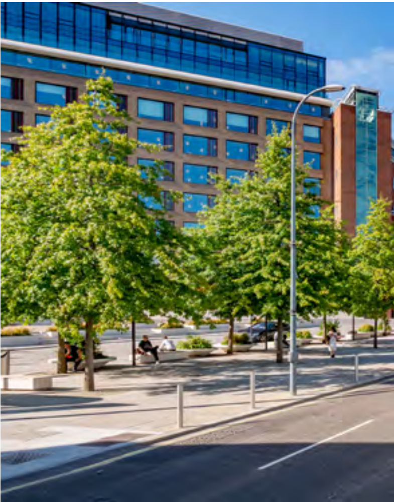
Completed installation of BBC Television Centre (Photographed in 2020)
