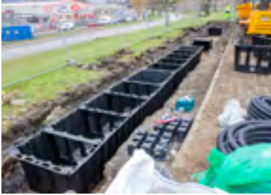
HydroPlanter can be installed in continuous, modular runs, or individually depending on site constraints and hydraulic performance requirements.
