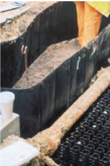
ReRoot 1000 installed to protect underground services and divert roots beneath pavement surfaces into the preferred rooting area.
