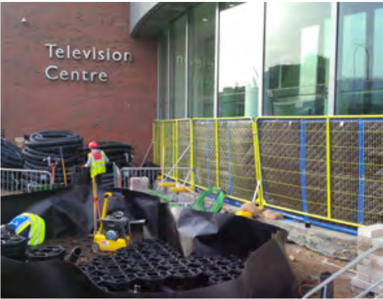
RootSafe will hold its form in a trench excavation. This makes installation quick and easy.
