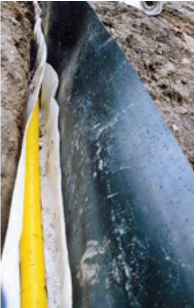
RootSafe can be used to keep tree roots from damaging services and paved areas.
