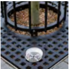
Inlet opens for irrigation.
