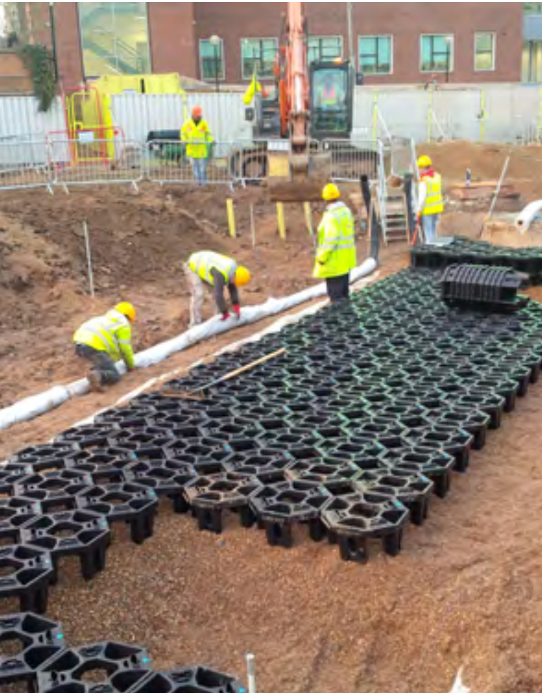
Installation of StrataCell soil cell system at BBC Television Centre, White City.
