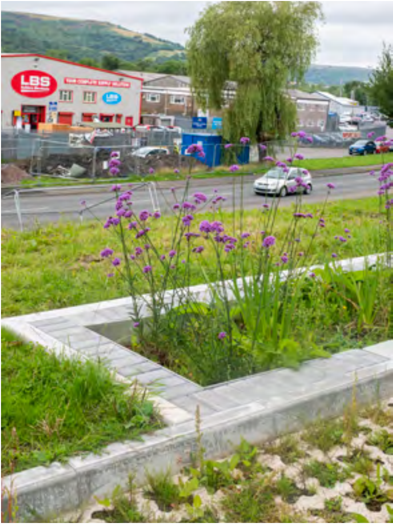
HydroPlanter can be installed in continuous, modular runs, or individually depending on site constraints and hydraulic performance requirements.
