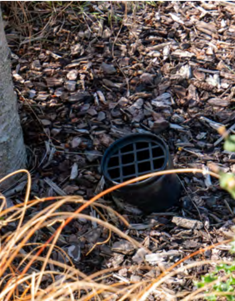
This illustrates the correct level for the RootRain Urban inlet. Too low could lead to blockages; too high can look obtrusive.
