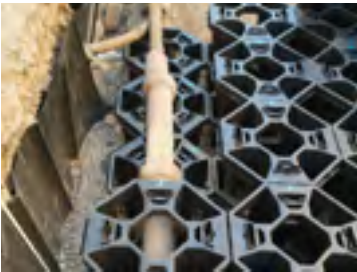
StrataCell is designed to work around below ground utilities and constraints.
