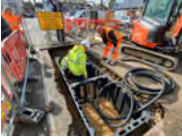
HydroPlanter can be installed in continuous, modular runs, or individually depending on site constraints and hydraulic performance requirements.
