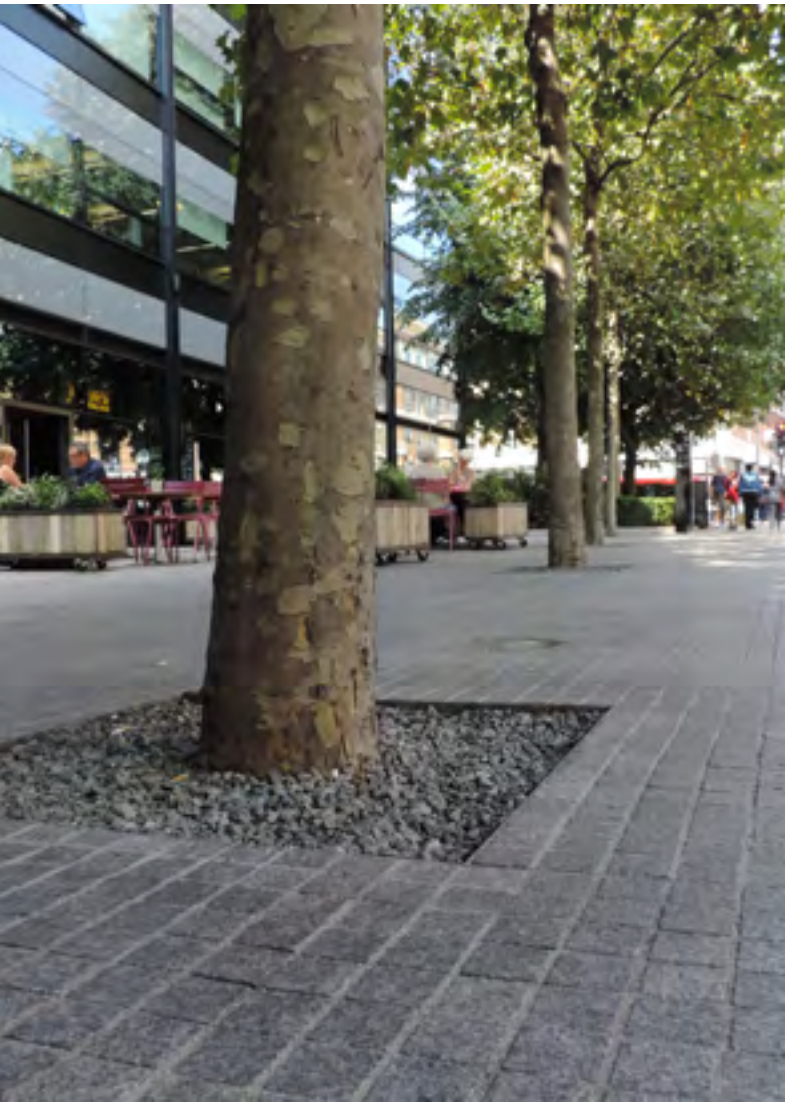
Very discreet concept allowing continuous paving over the tree pit.
